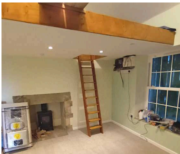
Completed hatch and ladder
