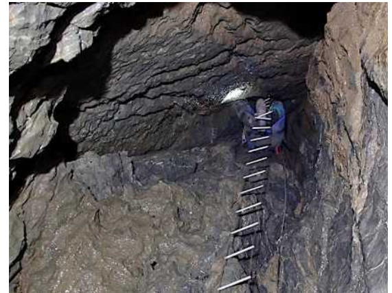
Eroded walls on the 11m pitch
