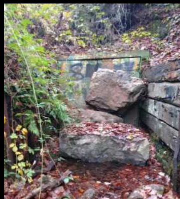
Entrance to adit now blocked with large boulders
