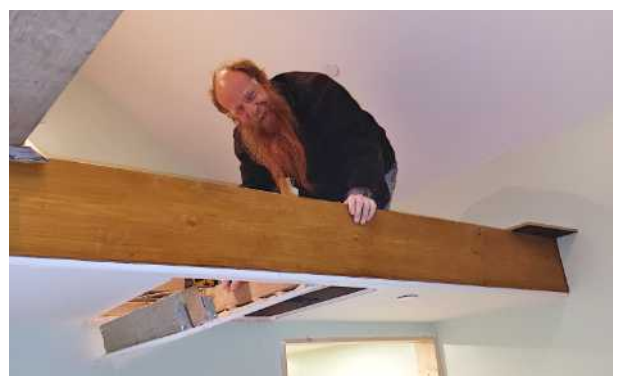
Cutting the access hatch for the mezzanine level
