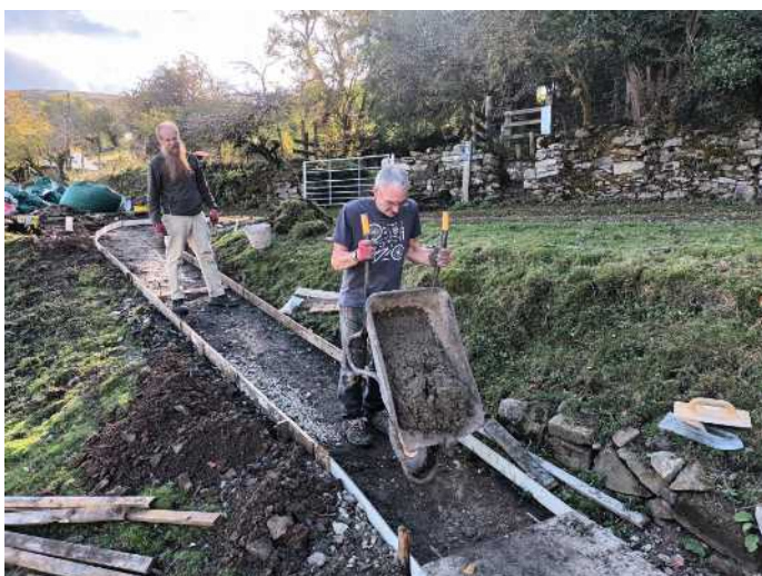
Andy and John laying the concrete path
