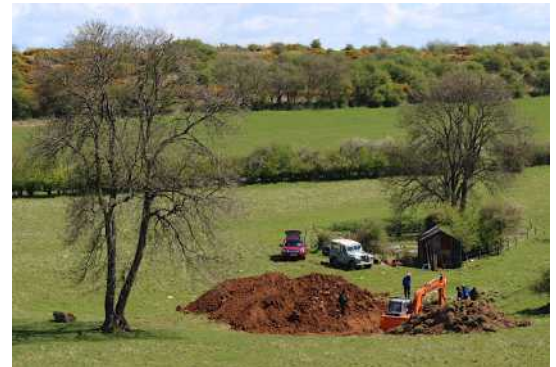
Start of the dig at Vurley
