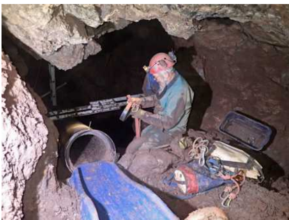
Spoil disposal shute into the main shaft's flooded depths
