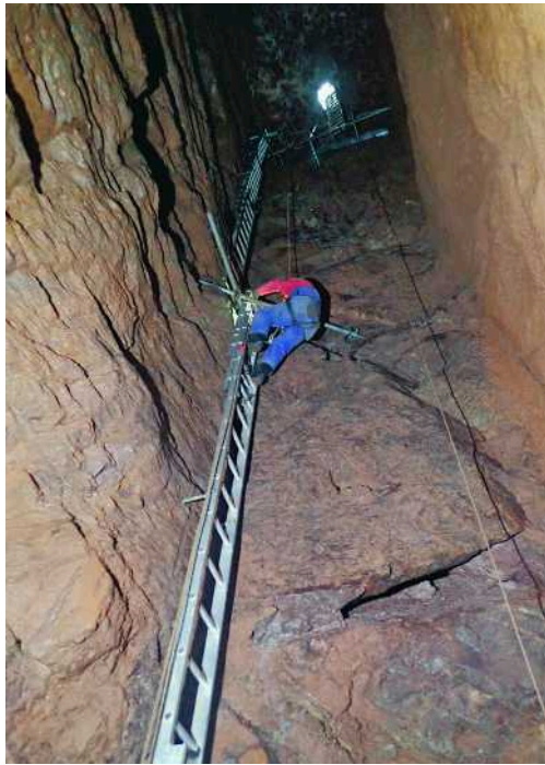
Switch over pole in the wet shaft. Traverse platform and cap above.
